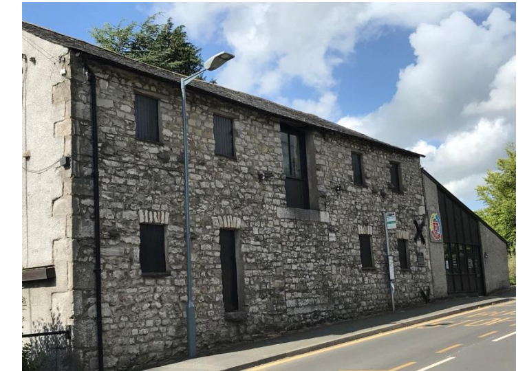
The Red Barn, Harmony Hill Milnthorpe c1750 was a bonded warehouse on the route that connected activities on the Port of Milnthorpe's estuary with the old main road which ran through Crooklands. In 1840 the barn was occupied by George Whittaker who made a fortune importing guano from South America for use as a fertilizer.
