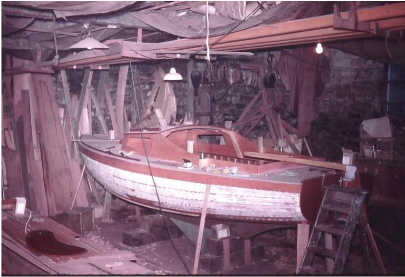
Hi Sheriff being built 1961
